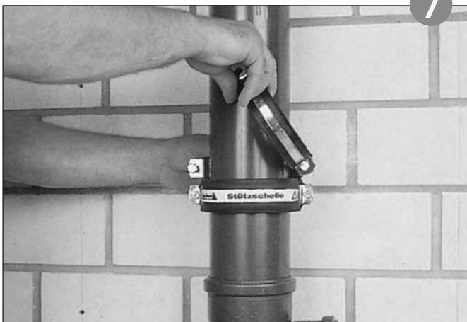
Fix the support ring onto the Friaphon pipe so that it rests on the support clip.
