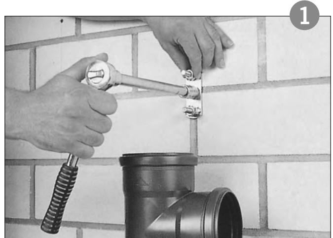
1 Mark, drill and fit the wall attachment.
