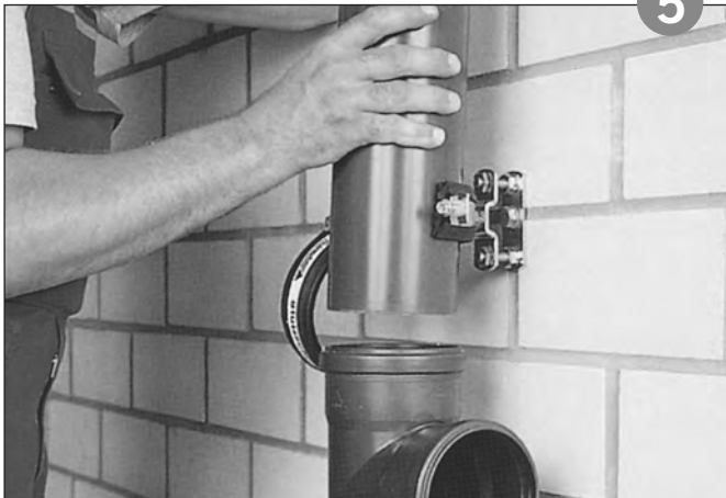
Open the snap lock of the support clip and insert the Friaphon pipe into the moulded fitting and clip fixer.
