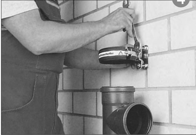
Fit the support clip to the wall attachment and tighten with a 17mm open ended spanner.
