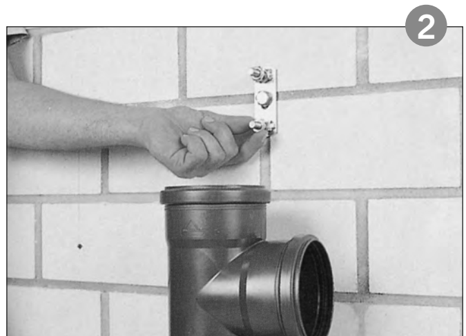
2 Adjusting the distance from the wall.
